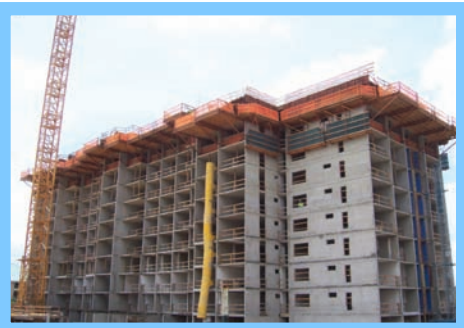
VC5™ replacing blanket-cure on high-rise project
