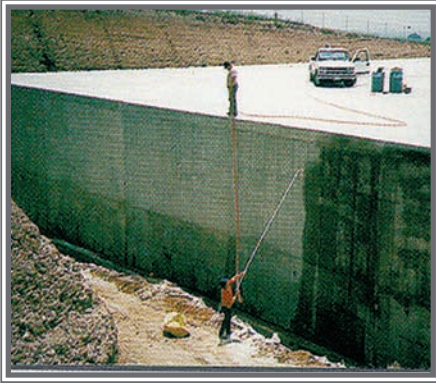
Water Tank; Laverne, California
